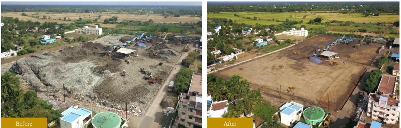
Image: Before and after images of a dumpsite reclamation project undertaken by Zigma in India to clear 15 acres of land from a 20-year-old dumpsite.
